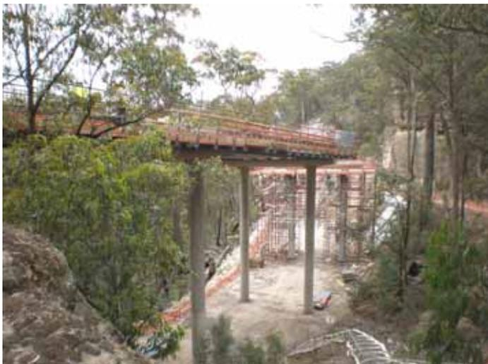
This stage includes major improvements, widening, realigning and sealing to the existing steep and narrow section from Bulee Gap to the Endrick River. The major earthworks and drainage structures are progressing well and traffic is being progressively switched onto the new alignment. A 1km length of new pavement was sealed in December 2008 near Billy's Hill.
